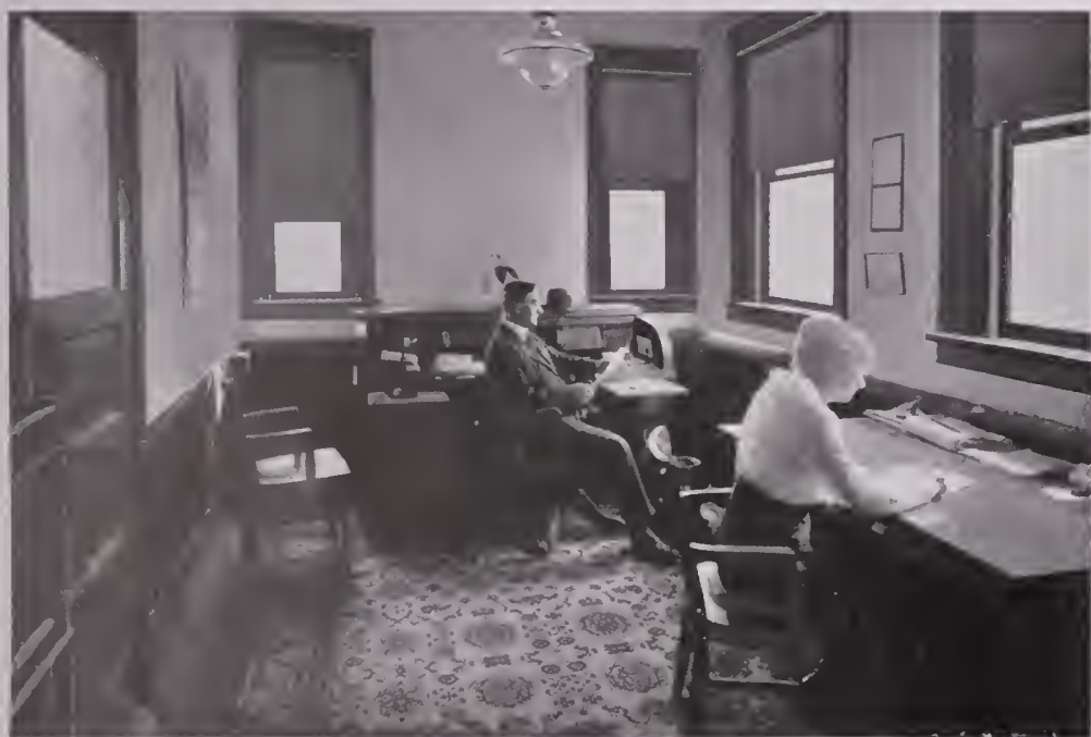
OFFICE OF GENERAL MANAGER DROP FORGE DEPARTMENT Drop Forge Office Building
